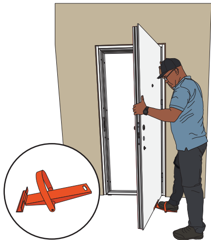
STEP 7. Fix the door frame (hinge side) to the wall using bolts.
